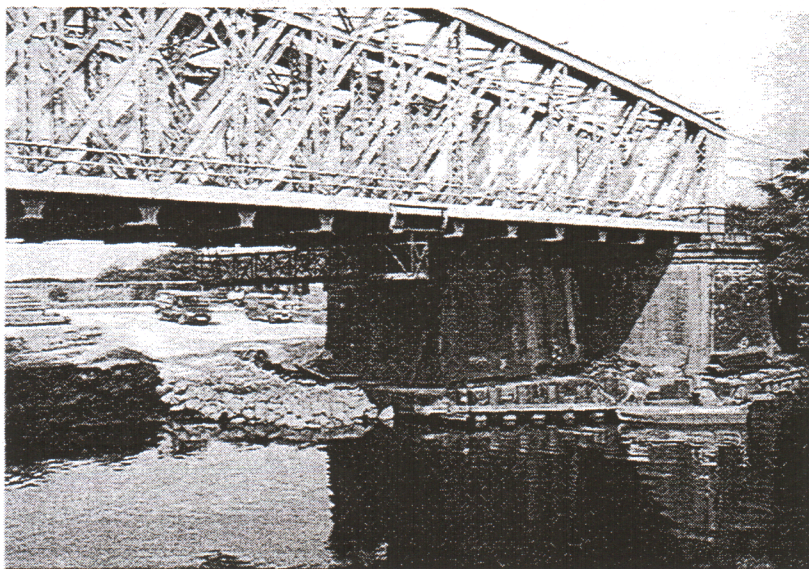
Fig.4 : The south-west pilecap prior to piling (view from river)
