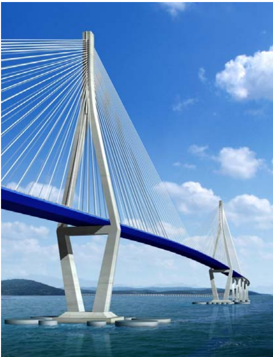
Fig. 3 Cable Stayed Bridge
