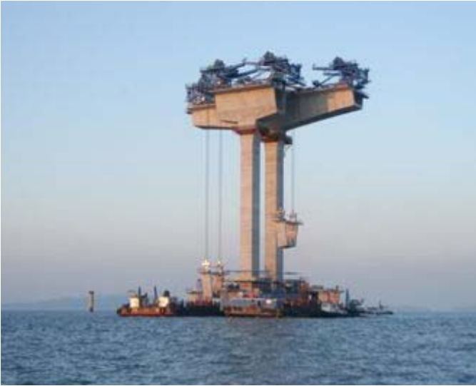
Fig. 5 Balanced cantilever construction
