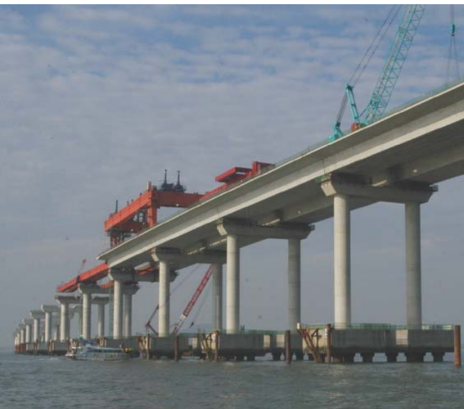
Fig. 6 Viaduct and launching gantry
